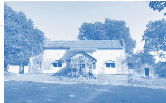
McCluskieganj, Conservation of Anglo India Estate - Conservation Project
